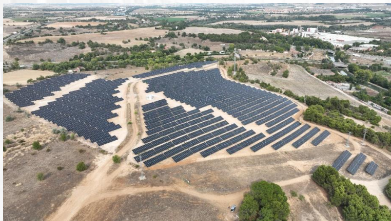
Industrial self-consumption PV installation on the ground. Lingotes Espaciales SA. Capacity of 5.9 MW. Finished in July 2024. Castilla y León.
