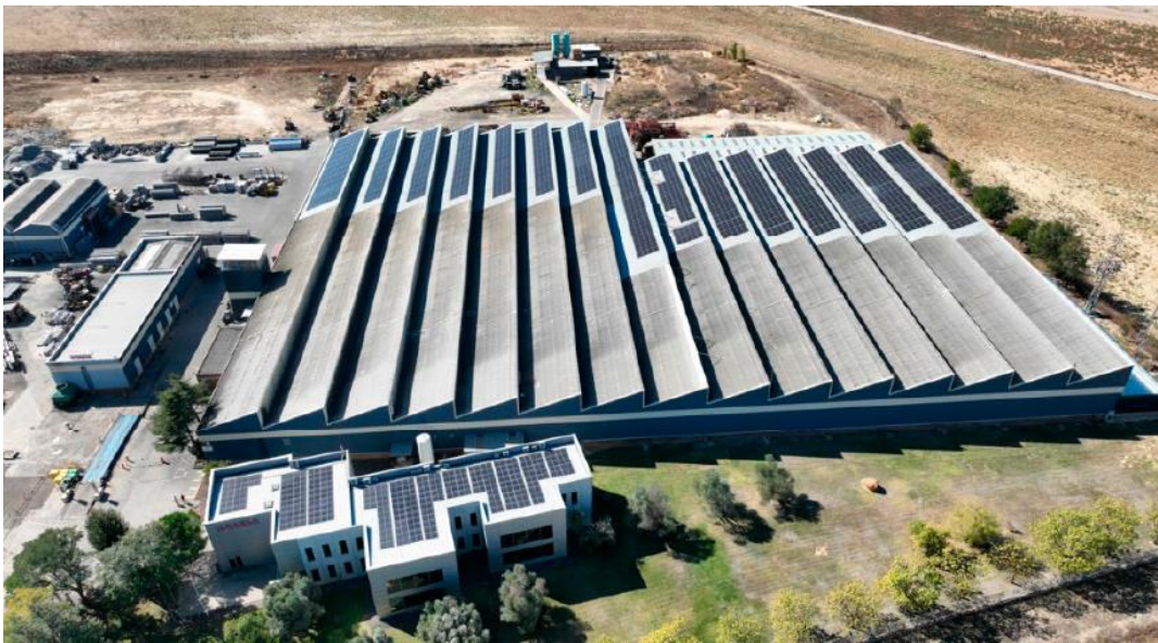
Riegos Agrícolas Españoles S.A. 800 KWp photovoltaic self-consumption plant in Castilla y León. Finished in April 2024
