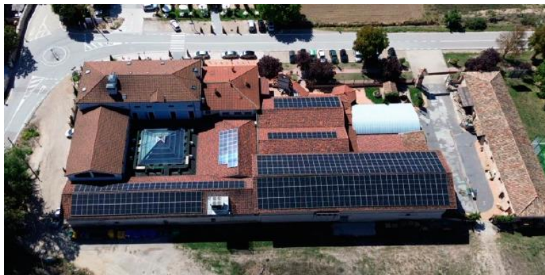
Bodegas Lagar de Isilla. 192 KWp photovoltaic self-consumption plant in Castilla y León.
